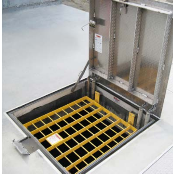
Improved floor opening
