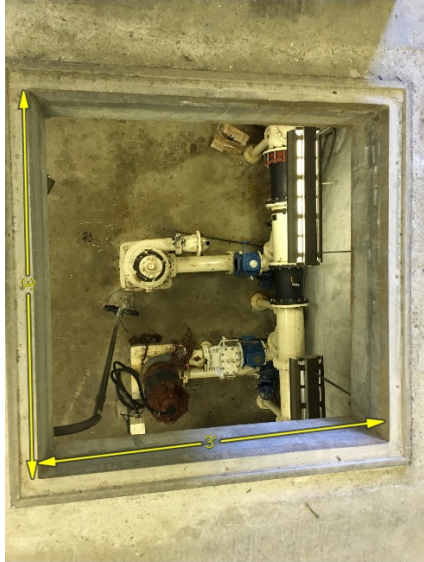
Existing floor opening
