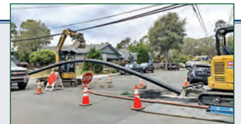
New line of pipe being installed on Isabella.
