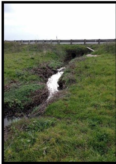
Figure 9.1: View facing southwest toward Drainage Ditch 2.
