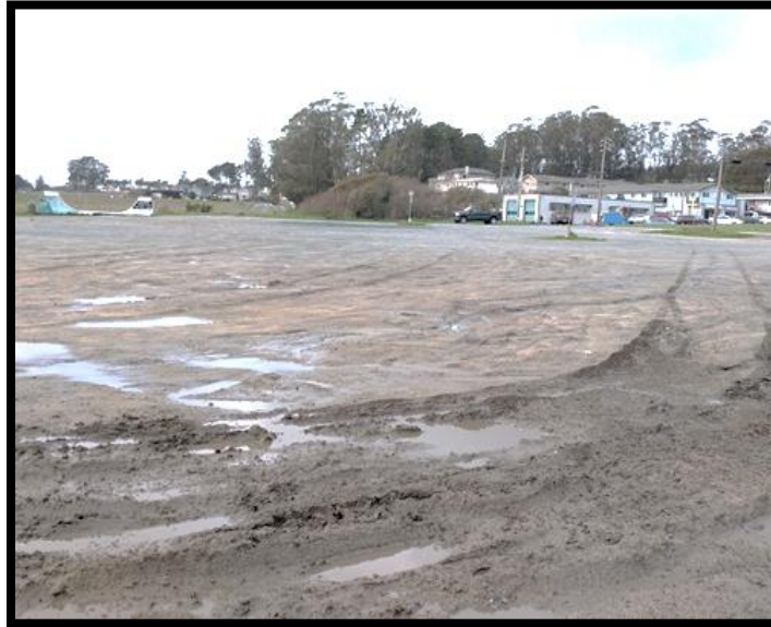
Figure 7.0: View facing northwest of the compacted area.
