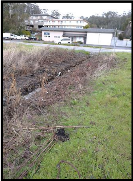
Figure 4.0: View facing north toward residential neighborhood of Ditch 1.
